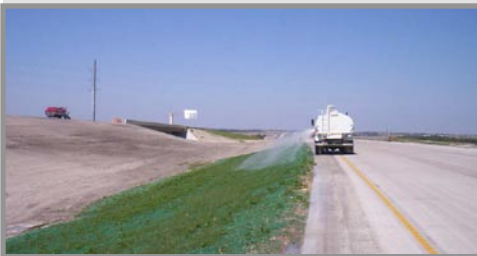
Finishing Touches in Segment 2
