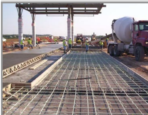
Ramp Toll Plaza Construction Near Elm Creek, Section 12
