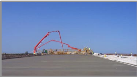
Bridge Deck Placement, Chandler Road Bridge
