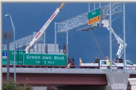
Signage Installation near the SH 45N/I-35 Interchange
