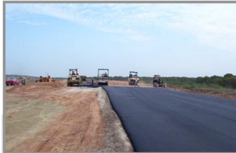
Ramp Toll Plaza Bondbreaker Operations Section 11
