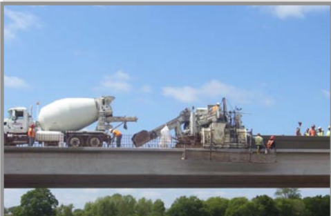
Placement of Concrete Barrier Rail, CR 109 Bridge
