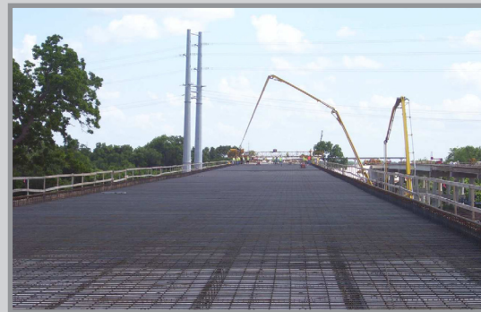
Bridge Deck Placement Colorado River Bridge, May 2007
