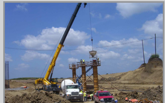
Bridge Column Construction Moore Road, June 2007
