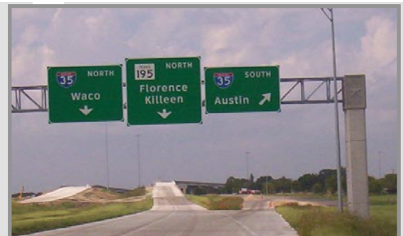
Signs Installed on SH 130 Segment 1 Near I-35 Interchange
