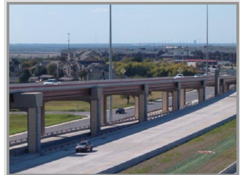
SH 45N Open to Traffic Just West of the I-35 Interchange
