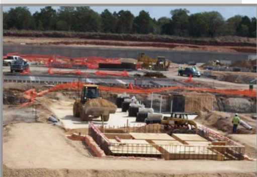
Mainlane Toll Plaza Construction in Segment 3
