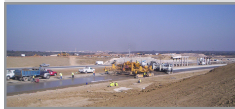
Paving Operations at Elroy Road
