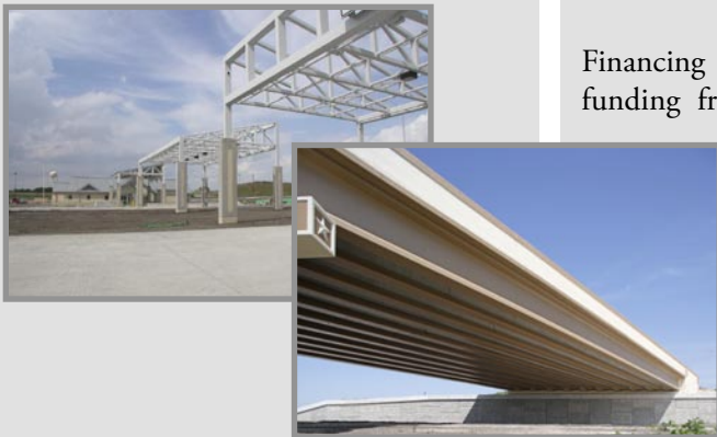
BELOW: SH 45N Mainlane Toll Plaza No. 2 at Wilke Lane
