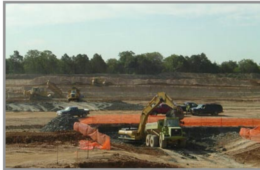
Tunnel Excavation for Mainlane Toll Plaza No. 7, Segment 3, Section 12
