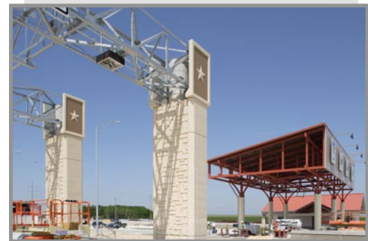
Mainlane Toll Plaza in Segment 2
