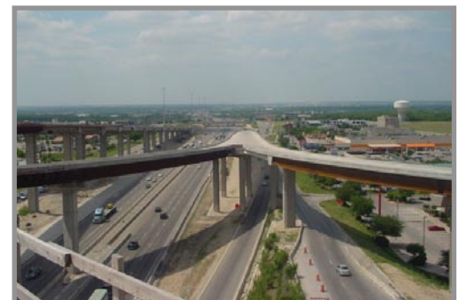
SH 45N/I-35 Intersection
