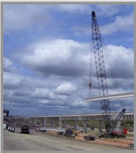
Bridge Beam Placement Operations at the Chandler Road Bridge, Section 4
