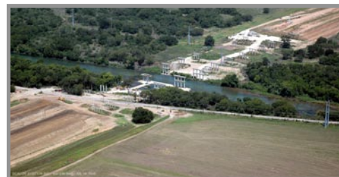
SH 130 at the Colorado River
