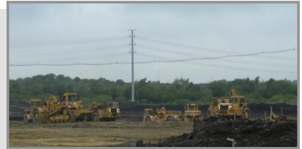
Excavation and Embankment Operations near Elroy Road
