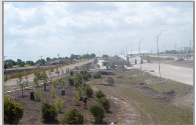
SH45N Mainlane Toll Plaza, Section 6, Looking East
