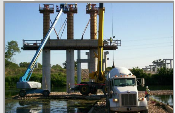
Construction of the SH 130 Bridge at the Colorado River
