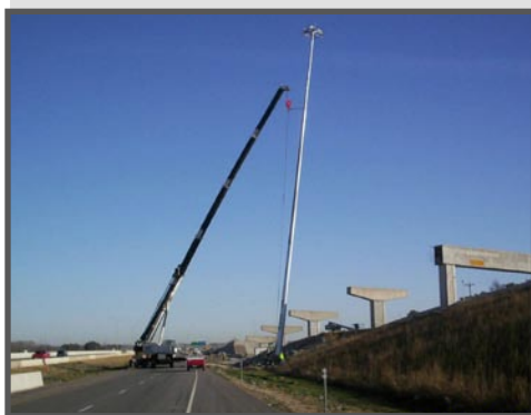
High Mast Lighting Being Installed at the SH 130/I-35 Interchange
