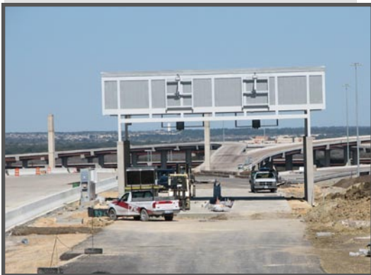
Ramp Toll Plaza, Loop 1 @ SH 45N, Looking North
