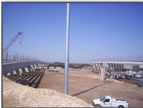
Installation of precast girders at the SH 130/I-35 bridges
