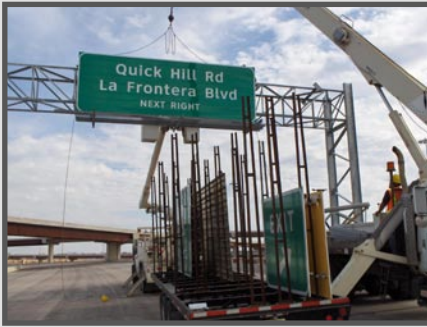
Overhead Sign Bridges, Section 3 (SH 45N/Loop 1 Interchange)
