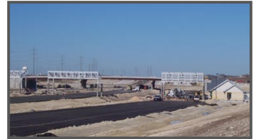
Mainlane Toll Plaza Construction, Section 6
