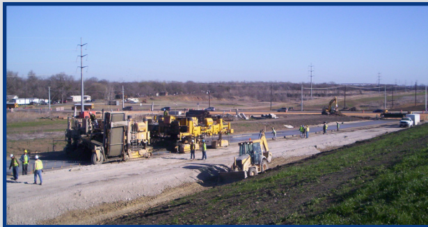
Paving South of Pearce Lane
