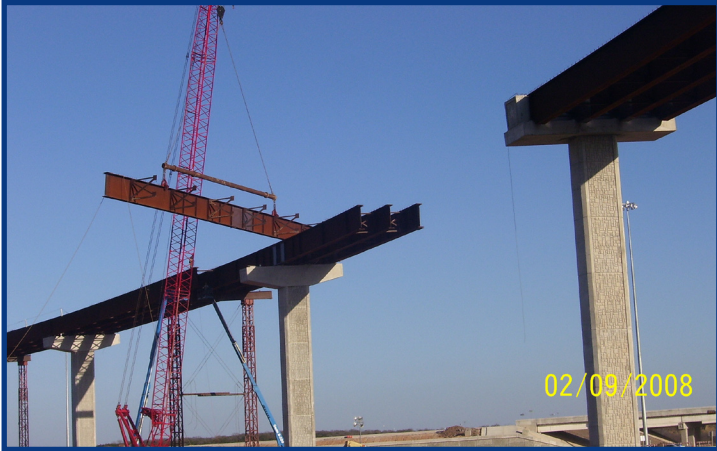
Steel Girder Placement at SH 71
