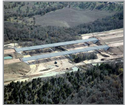
SH 130 at Decker Creek, Segment 3
