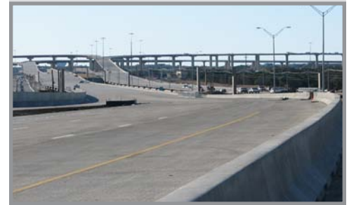
SH 45N at US 183, looking west toward the Interchange
