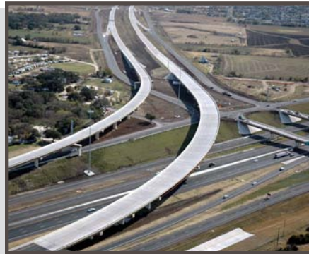
SH 130 at I-35, Section 1
