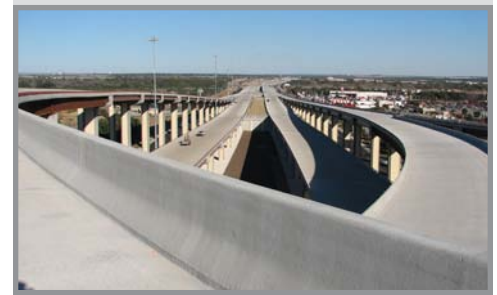
SH 45N at US 183, looking east from the Interchange
