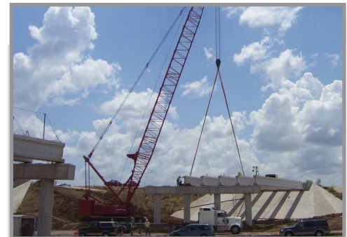
Concrete Beam Placement at Pearce Lane
