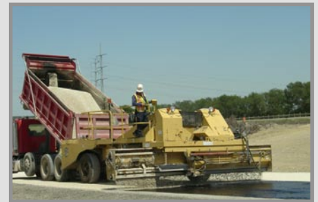
Sealing the Temporary Portion of the FM 973 Detour, Section 11
