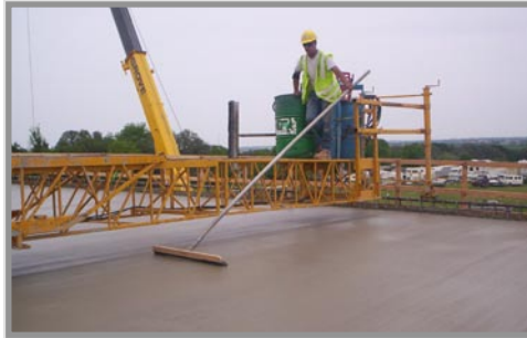
Bridge Deck Finishing, SH 130 @ I-35
