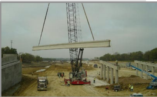
First Beams Set in Segment 3, FM 973 Bridge, Section 11
