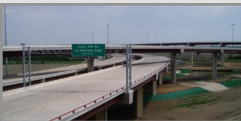
SH 45N/Loop 1 Interchange
