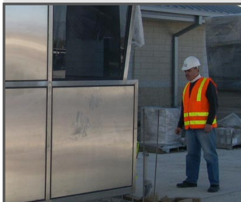
Tony Alam, Meta-Lite, Inc., supervises off-loading and installation of toll booths
