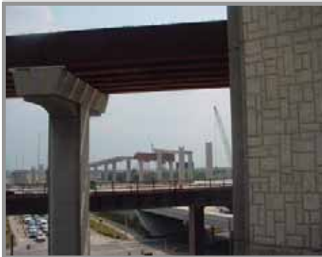
SH 45N @ US 183, Section 8, Looking South
