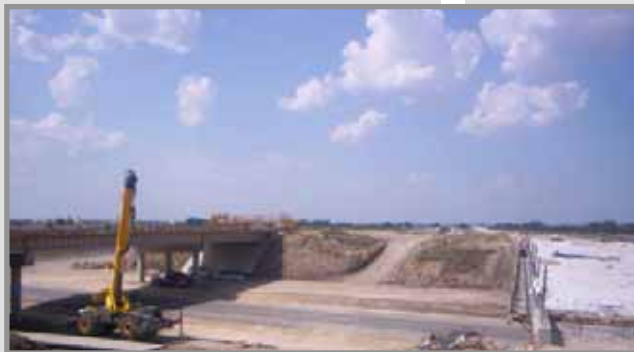
SH 130 @ CR 152, Looking North
