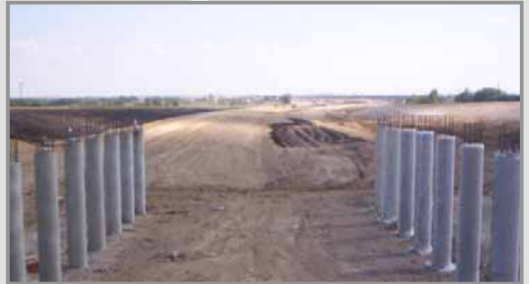
SH 130 @ SH 29, Looking South
