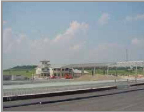
Mainlane Toll Plaza, Loop 1
