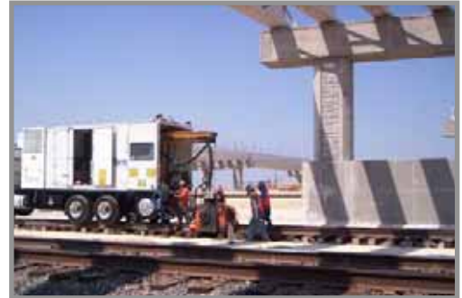
Welders working on "shoo fly" construction, SH 130 @ US 79
