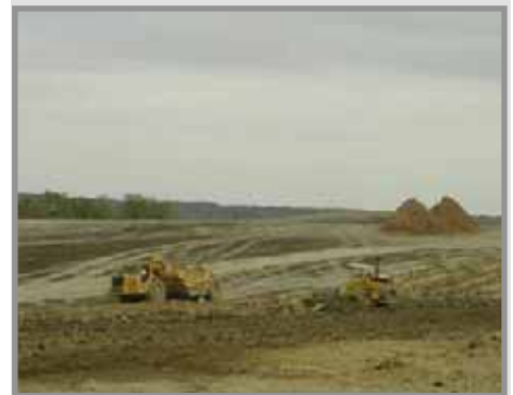
Embankment work near Blue Bluff Road, Segment 3, Section 11
