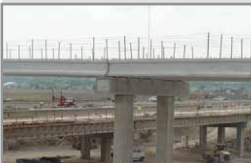
Construction of the SH 130 bridges over US 79
