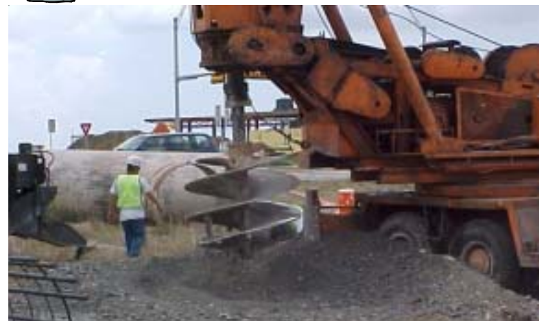
Bridge foundation shafts being drilled at the La Frontera intersection (Section 4).
