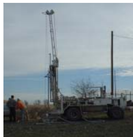
Geotechnical field exploration and sampling work being conducted on SH 130.
