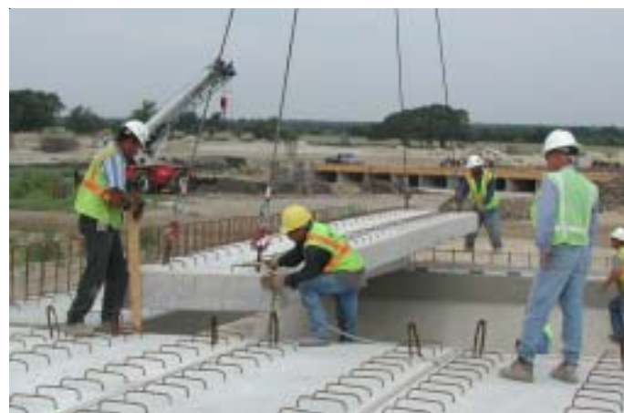
Precast deckform panels being placed in preparation of the bridge slab placement (Section 3).
