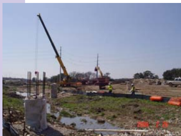
Drilled shaft construction along Loop 1
