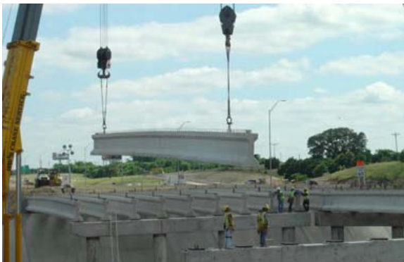
120' beams placed at Berry Creek Bridge
