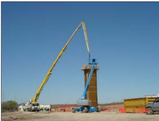
Column placement at SH 45N/SH 130 Interchange
