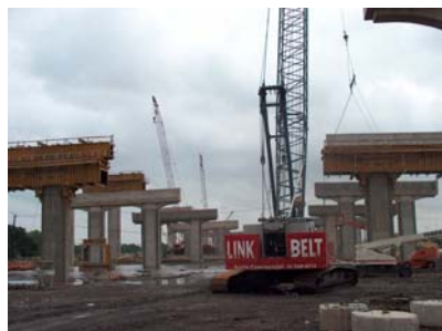
SH 45N - Section 8 looking east
