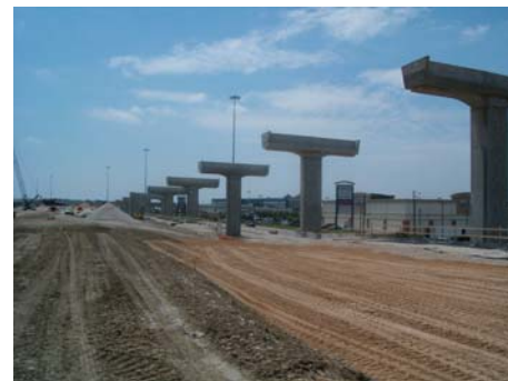
SH 45N southbound/ westbound direct connector - Section 4
