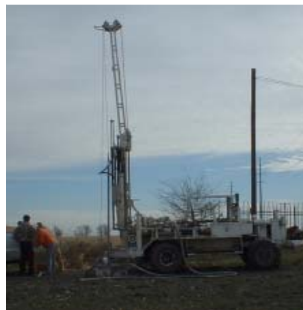
Geotechnical field exploration and sampling work being conducted on SH 130.
