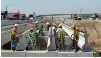
Dry Berry Creek--delivery, unloading, and setting beams
