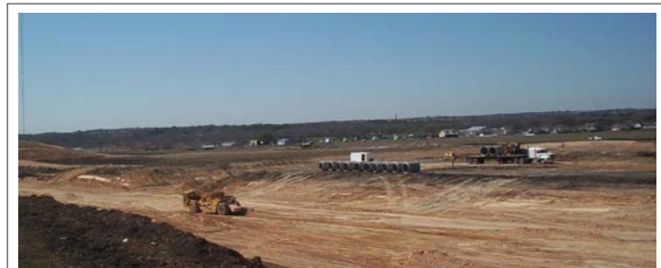
SH 130 Earthwork in Section 5
