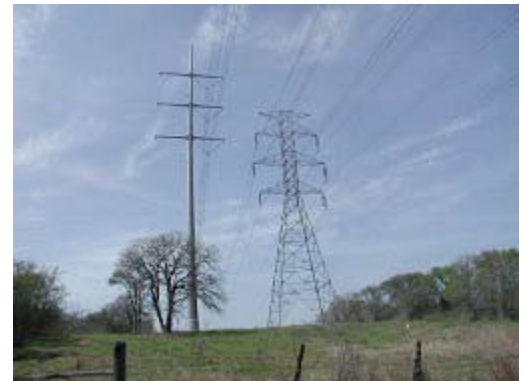
Electric transmission lines spanning SH 130 proposed ROW
