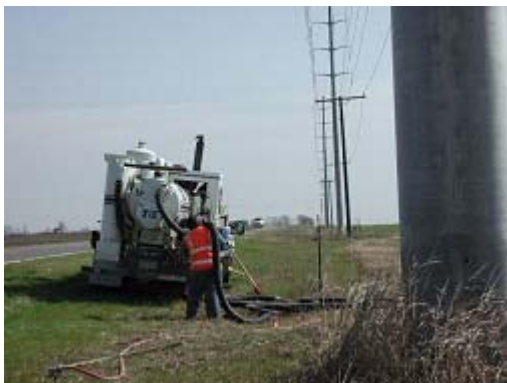
Subsurface utility work identifying crossings on SH 130
