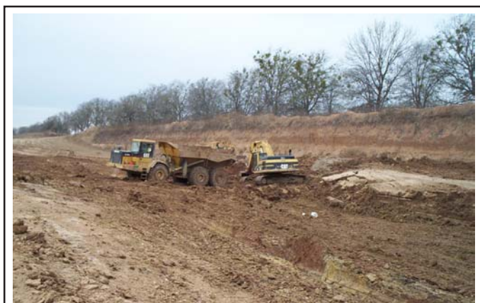
Figure 5 Mud Removal in the North Pit near FM 973
